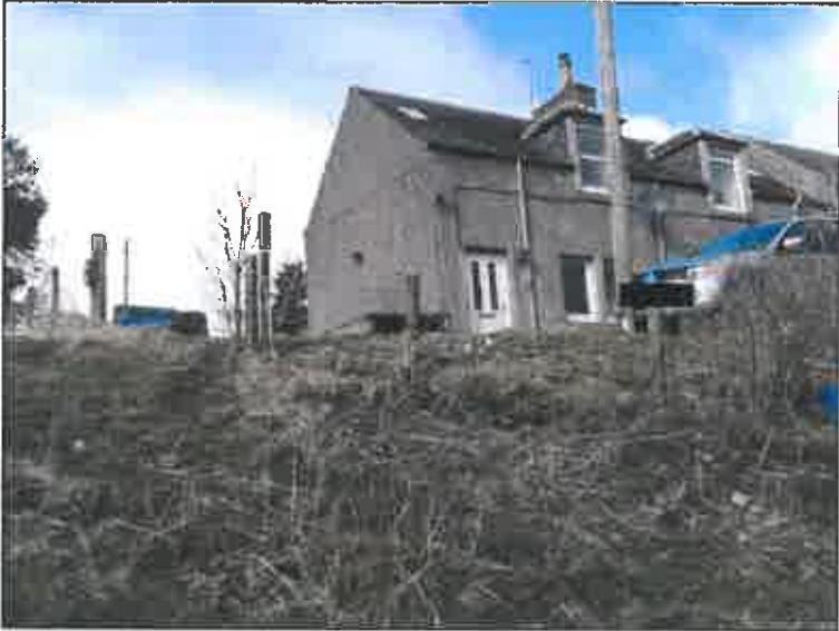
Fig 8: View of southern elevation
