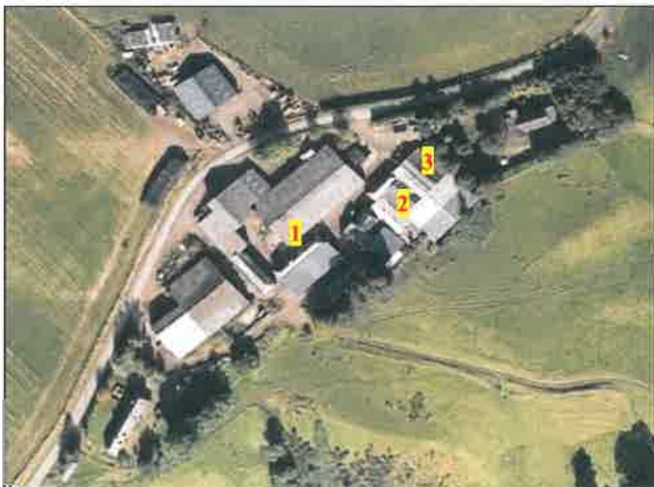
Fig. 1: Aerial Photograph of Wormiston Farm Buildings showing location of the 3no. traditional buildings in the heart of the farm
