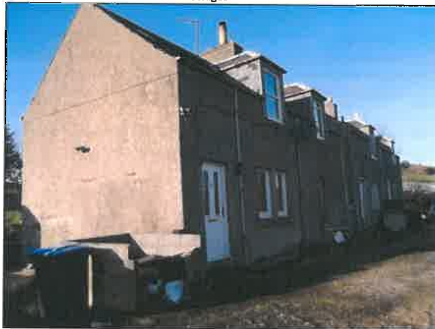
Fig. 9: East elevation of Wormiston Cottages
