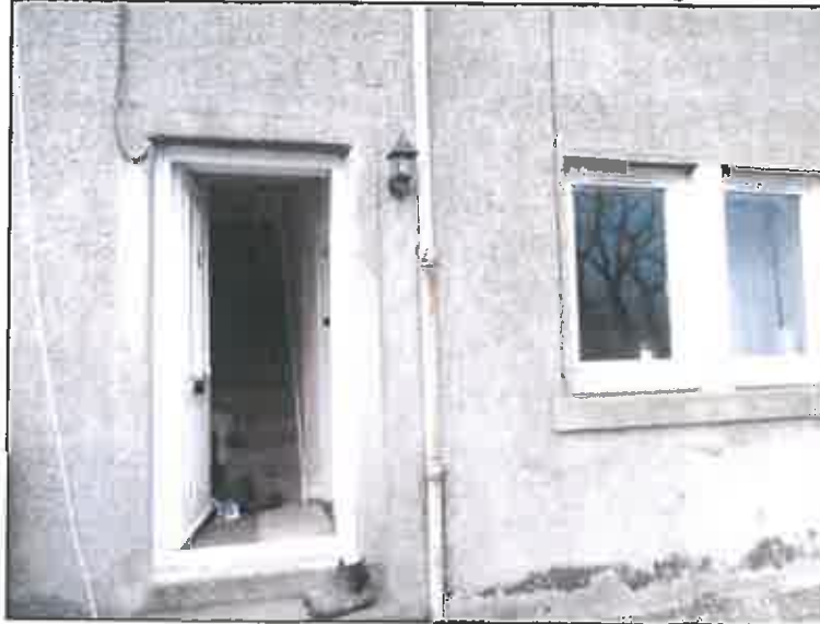
Fig 2: Entrance to 3 Wormiston Cottages with steep and narrow flight of stairs:
